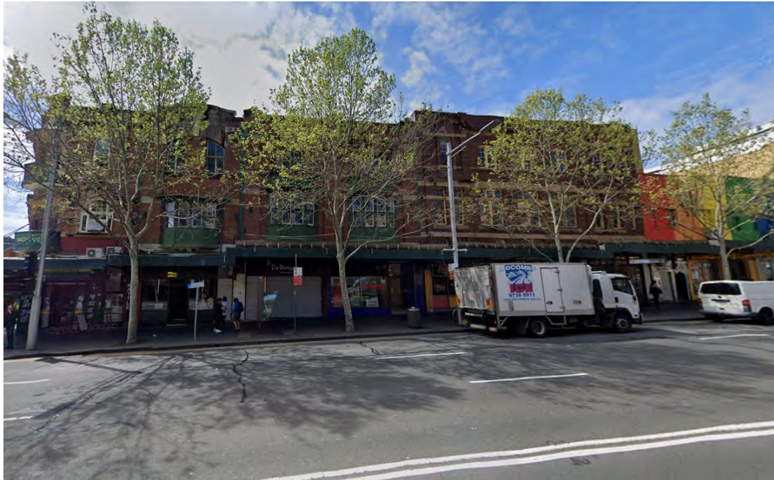
Figure 13 – View of Group 3 buildings (Source: Google Streetview).
