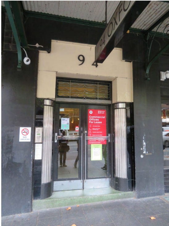
Figure 5 – View of entrance to 94 Oxford Street.
