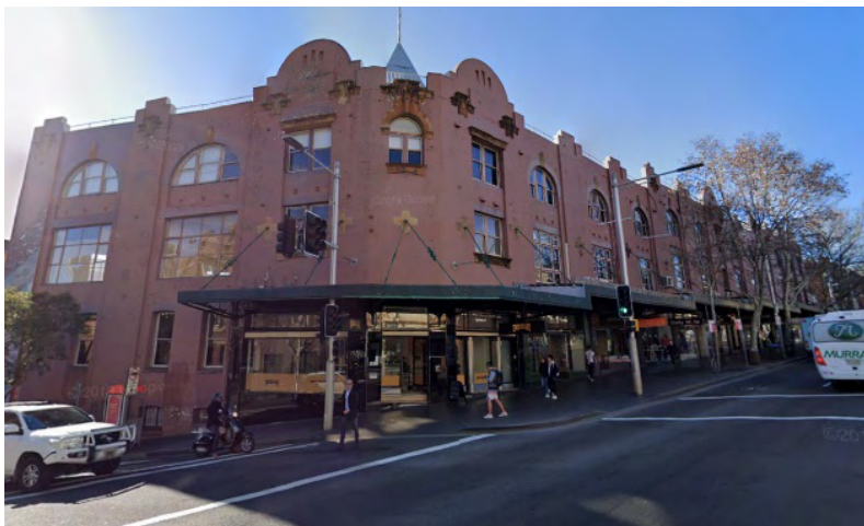
Figure 3 - Exterior view of group 2 building at 82-106 Oxford Street, showing the Oxford and Crown Street facades. Source: Google Streetview
