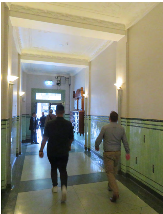
Figure 7 – View of entrance foyer at 94 Oxford Street showing tiled dado, terrazzo floors, pressed metal ceilings and Inter War lighting.
