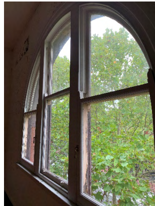
Figure 12 – Typical second floor window on north wall of 94 Oxford Street.
