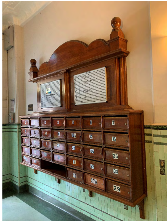
Figure 6 – View early tiles and timber letterboxes within entrance foyer of 94 Oxford Street.
