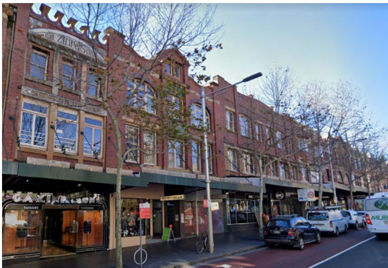
Figure 1 - Exterior view of group 1 buildings at 56-76 Oxford Street, showing buildings at the western end of the group. Source: Google Streetview.
