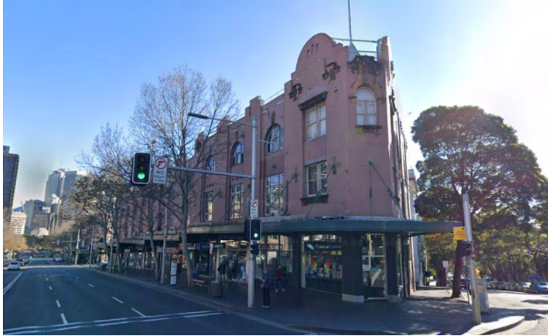
Figure 4 - Exterior view of group 2 building at 82-106 Oxford Street, showing the building façade at the corner of Oxford and Palmer Street. Source: Google Streetview
